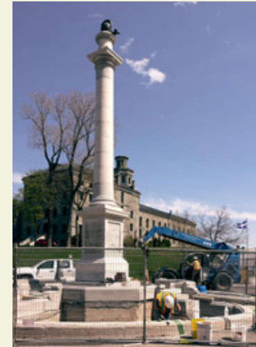
Restoration work of the Wolfe Monument
